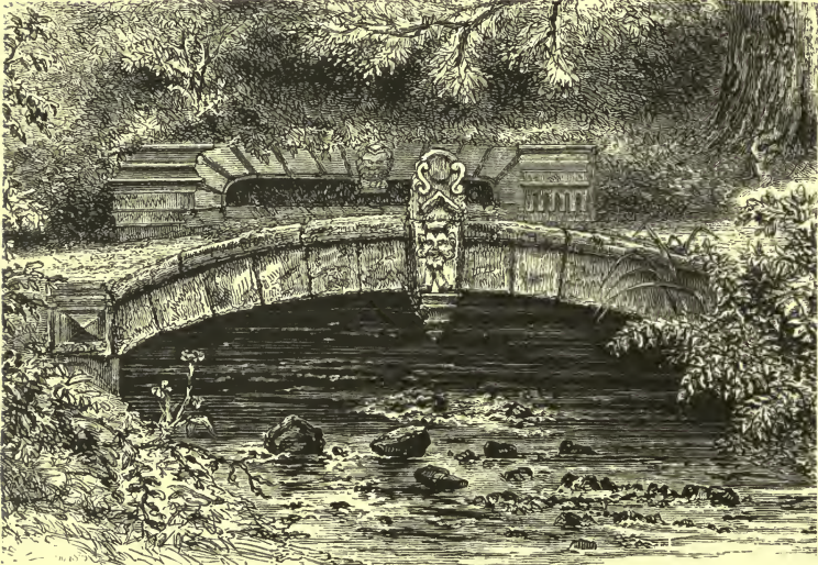
BRIDGE MADE OF STONES SAVED FROM THE OLD PARLIAMENT HOUSE.
